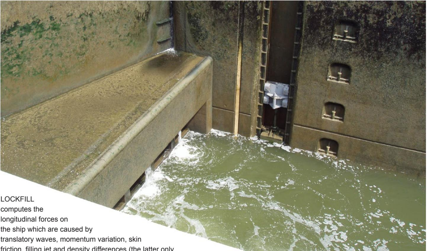
Figure 3 Levelling through culverts of the new lock at Panheel (NL).
